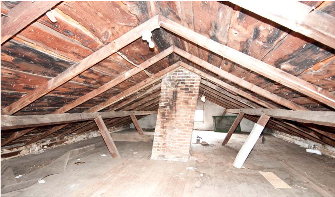
Garret, main block, looking north
