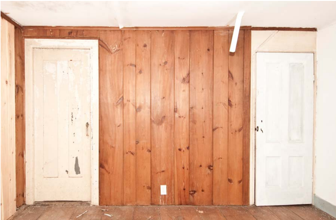
Southeast chamber, south wall
