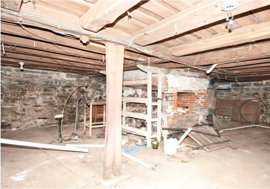
Basement looking northwest
