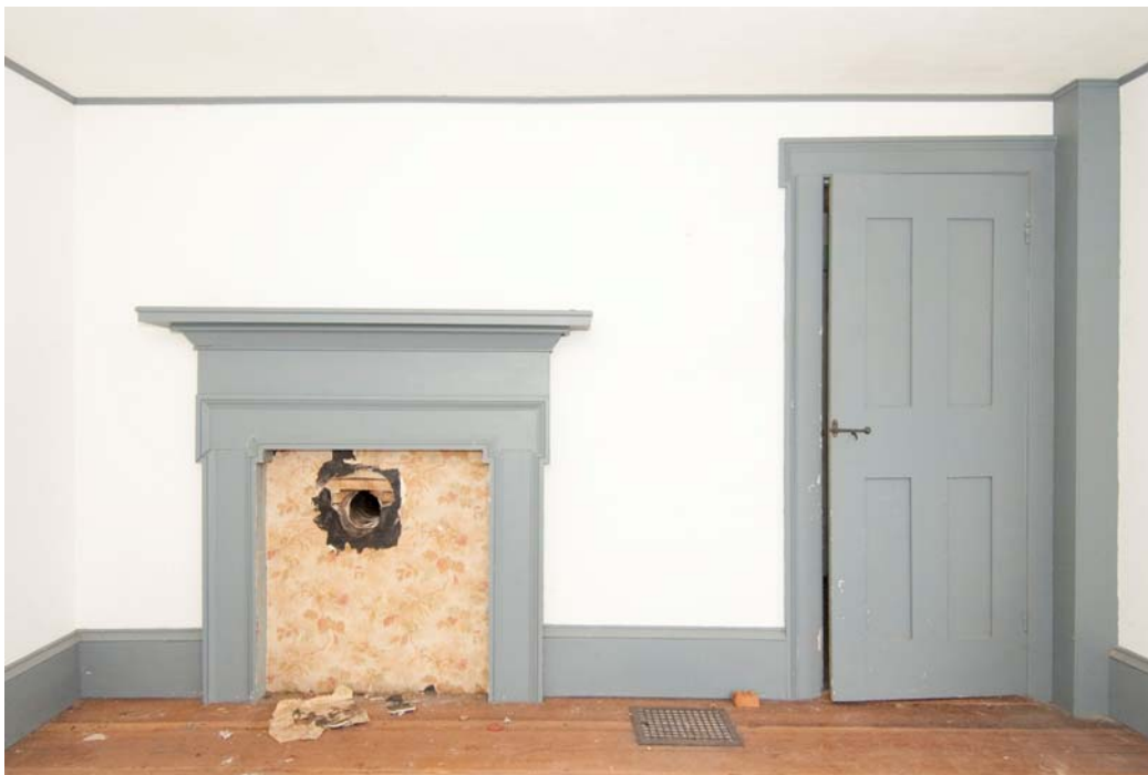
North parlor, south wall
