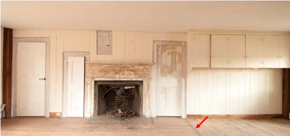
South room, north wall, arrow indicates location of earlier partition
