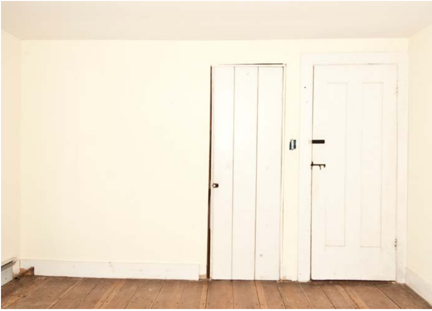
Northeast chamber, south wall
