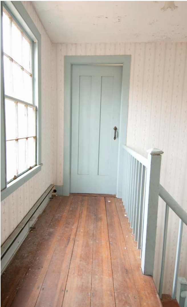
Stair hall, second floor, looking north
