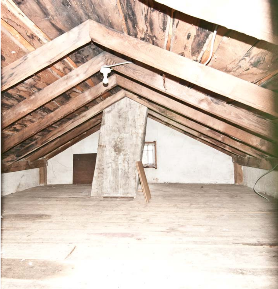
Kitchen wing garret, looking south
