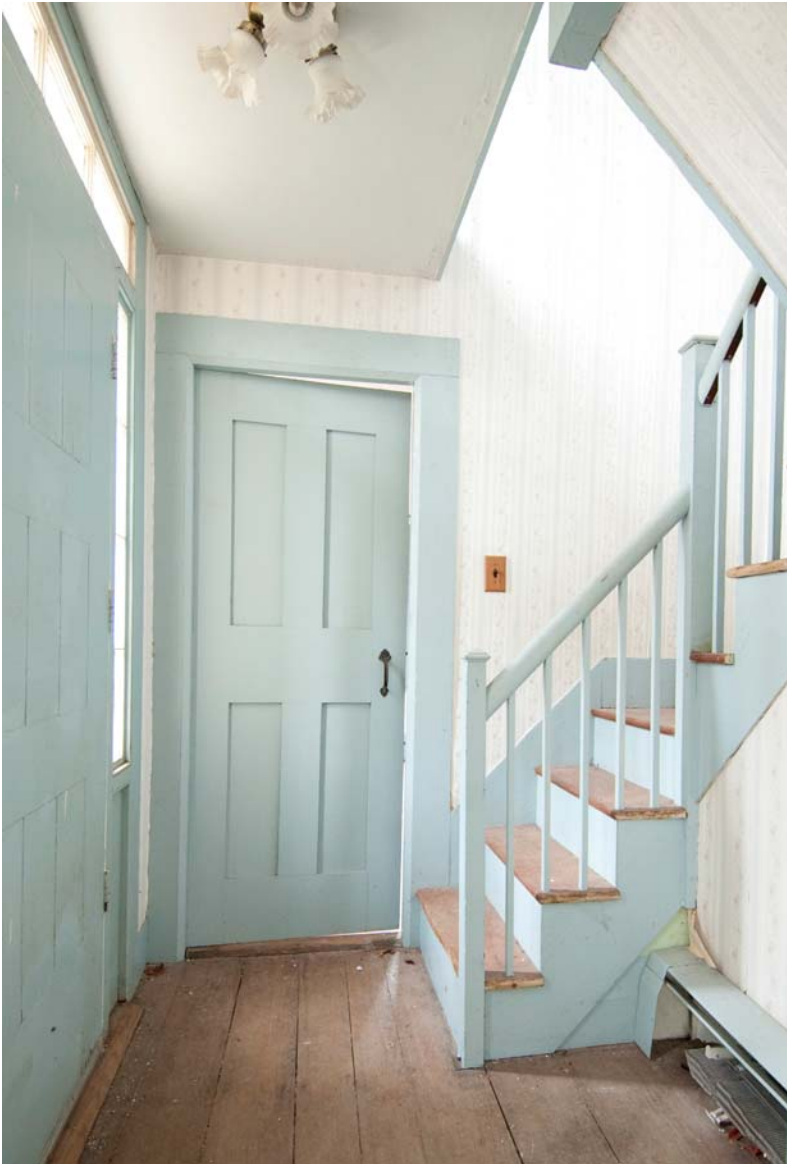
Entry looking north
